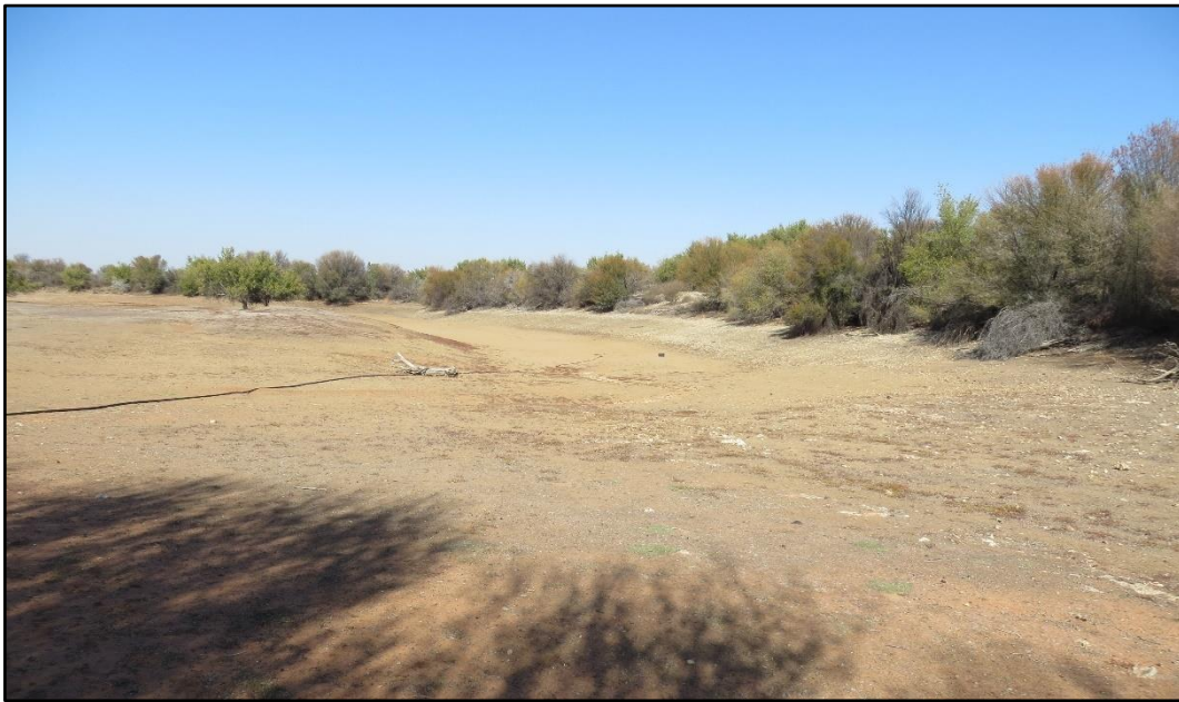
Plate 10: Completely dry dam on the Doringdam Spruit.
