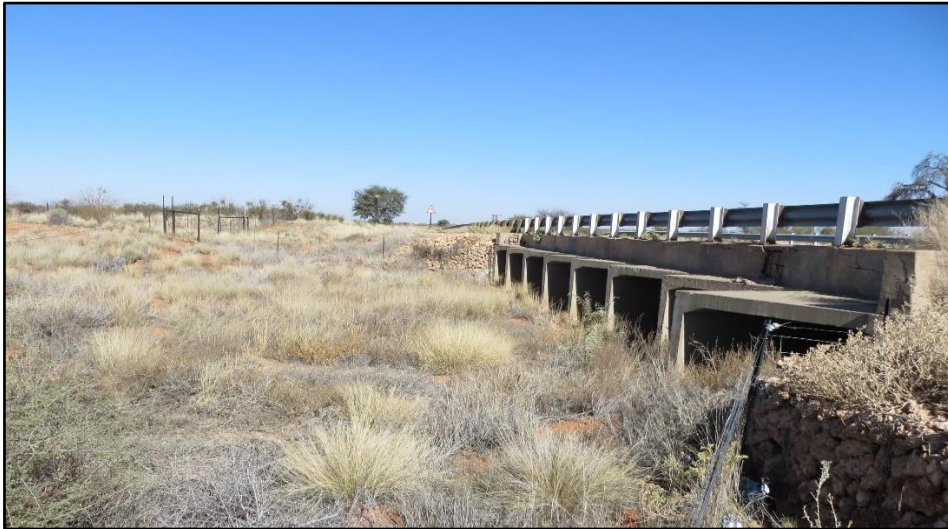
Plate 9: Road R360 bridge over the Doringdam Spruit showing the large culverts
